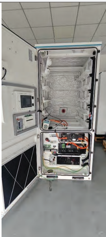
Internal view – Open doors
